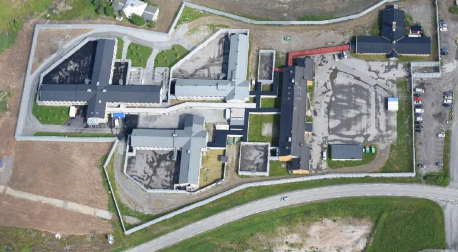
Aerial view of Trandum Detention Centre (National Police Immigration Service)
